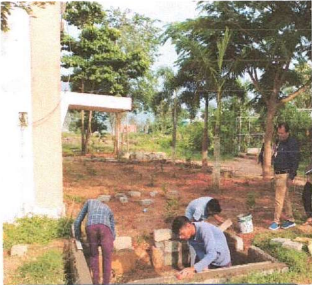
Water Harvesting Pit during Construction
